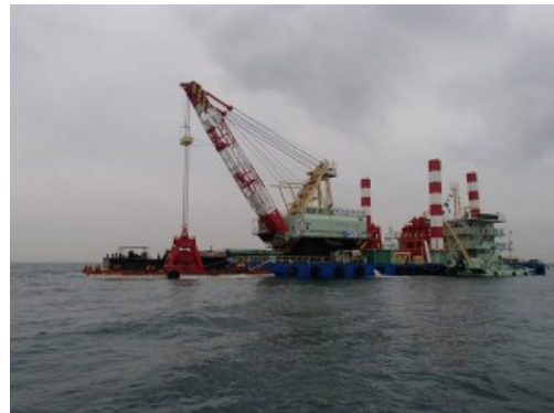
"Wakawashi Maru" grab dredging construction
