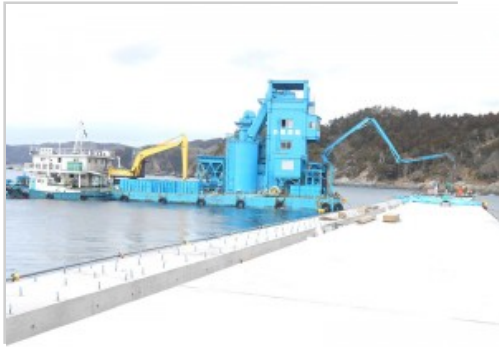
"Concrete mixer ship" concrete placement work
