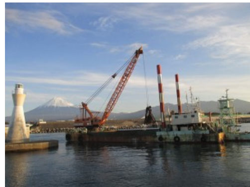
"Ryuo" grab dredging construction
