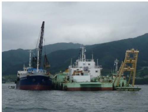
"WTS-1000" Spread sand construction
