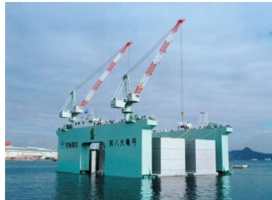
No.8 Taiki go: Caisson work platform
