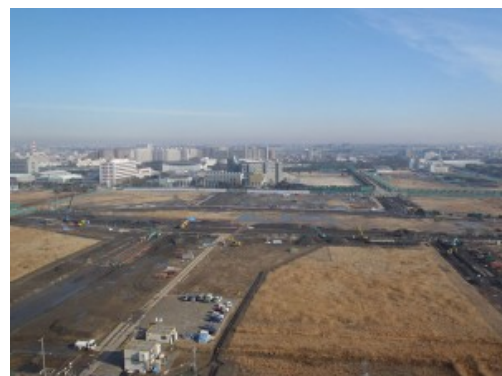
Sewerage and construction work
